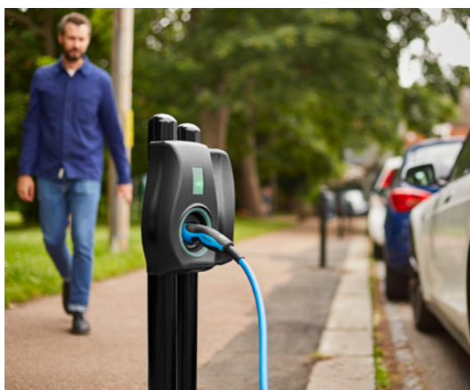
◀ A chargepoint on a residential street.
