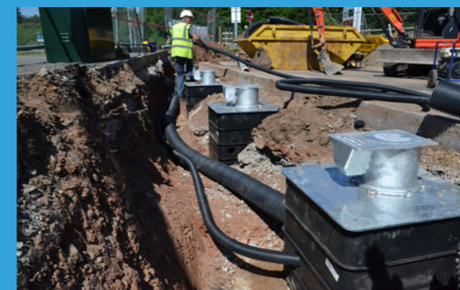
Civils infrastructure being installed
